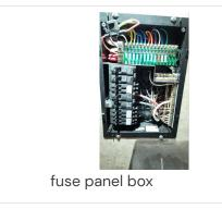
(2) Inspector observed 2 wires under the 12v lugs. It is recommended that this be evaluated for repairs by a qualified RV technician.
